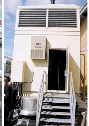
Left: photovoltaic system on the Horse Palace roof. Right: trigeneration plant at the Direct Energy Centre provides heating, cooling and 1.6 MW of electricity.
