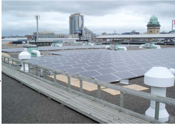
Left: photovoltaic system on the Horse Palace roof. Right: trigeneration plant at the Direct Energy Centre provides heating, cooling and 1.6 MW of electricity.
